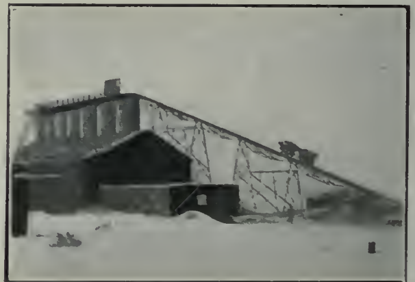
"Standard" Hydrating Plant, Guelph, Ont.
